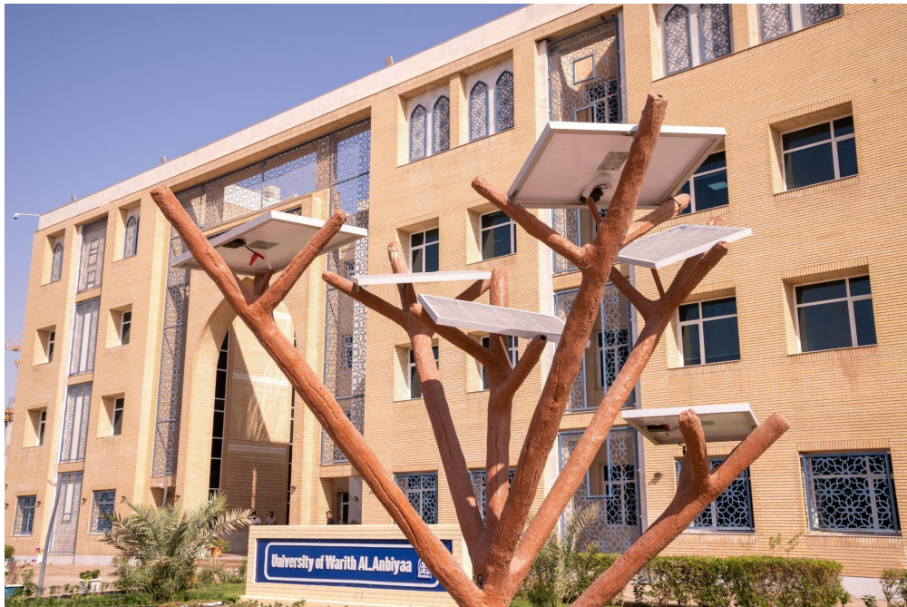
A single Solar panel tree among others for charging
