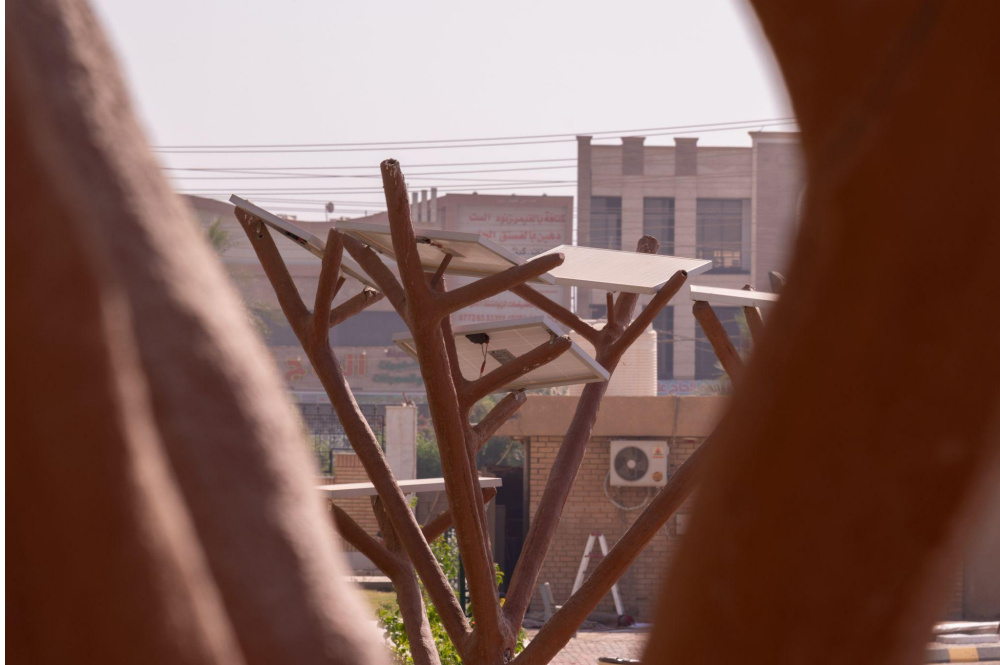
Decorative trees with solar panels
